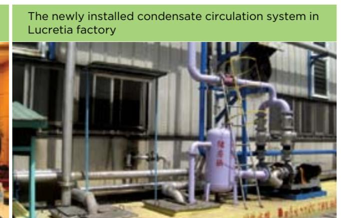
The newly installed condensate circulation system in Lucretia factory
